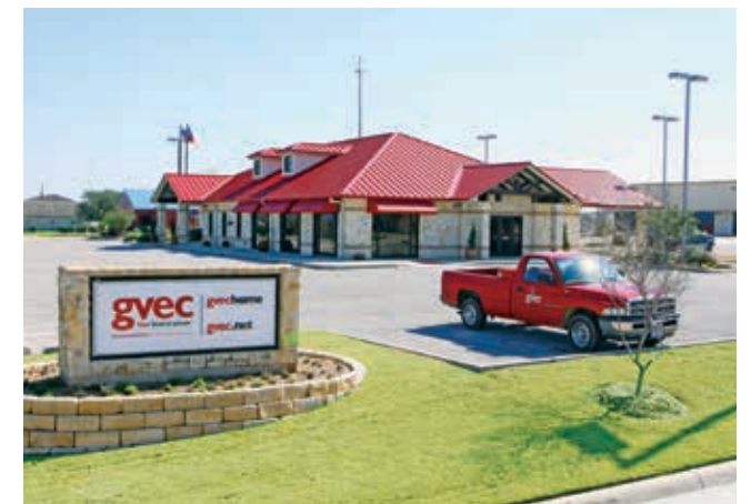
Spurred from proactively planning for growth in the western region of the service area, the La Vernia office was opened in October 2005 at 13849 U.S. Highway 87 West, complete with a GVEC Home appliance showroom.
