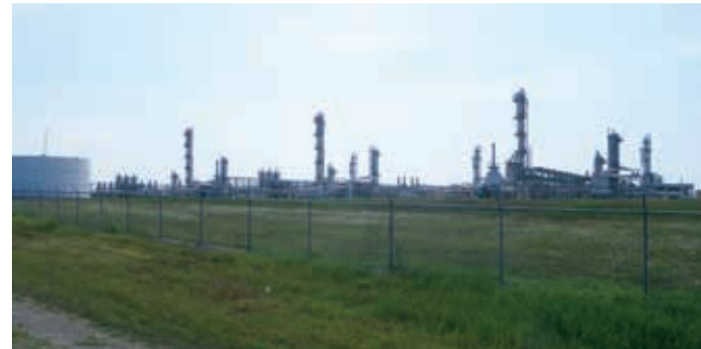
Enterprise Partners' natural gas processing plant in Yoakum came online in 2012. It is just one example of the large oil-and-gas-related electric loads GVEC has supported since the discovery of the Eagle Ford Shale in 2008.
