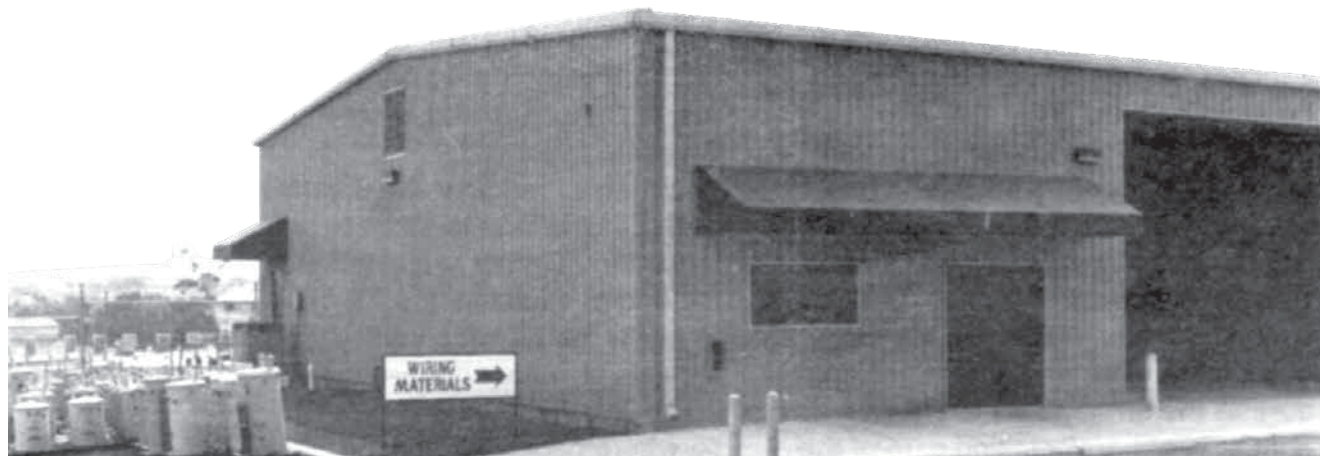
Since the early years, the GVEC Resale Shop provided electrical supplies, wiring materials, and recommendations for safe projects to the public. Located both in Seguin (at the Area office) and in Gonzales, a new location was opened in 1995 off Oakland Avenue, just behind the Gonzales office off Sarah DeWitt Drive. Today, this area houses GVEC.net operations.
