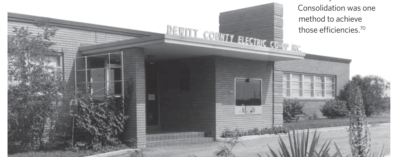
The DeWitt County Electric Cooperative, more informally known as the DeWitt Electric Cooperative, was established at the same time as GVEC and served a close, but much smaller member base. This made the cooperative a prime candidate for a merger with GVEC which would result in savings for all area cooperative members.
