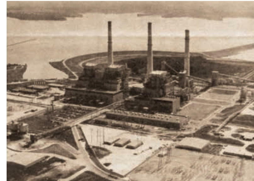
The Fayette Power Project was a joint effort of the Lower Colorado River Authority and the City of Austin. Electric energy produced at the generating plant provided more than 91 percent of the wholesale power purchased by GVEC at the time of its fifteen-year anniversary in April 1994.
