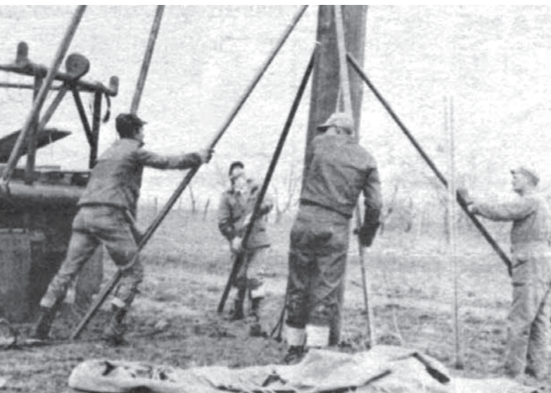
Every step of line work in the early years was manual as these GVEC linemen in 1953 demonstrate.
